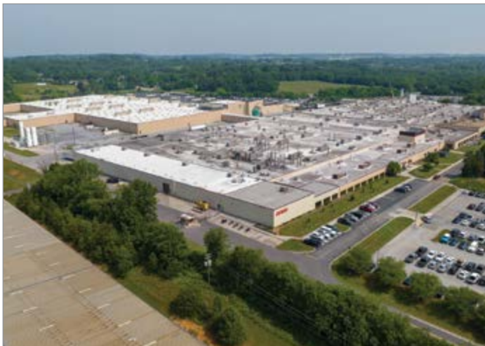
A compressed air leak management program generated excellent results at DENSO's Maryville, TN, manufacturing facility.
