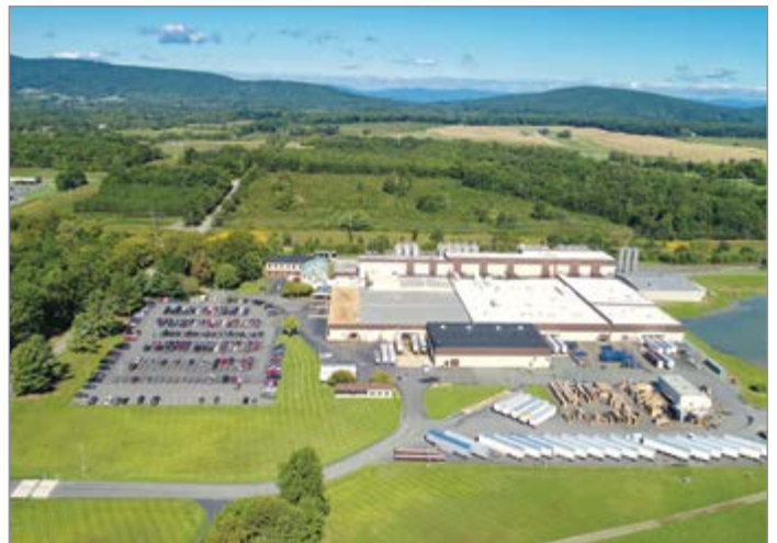
An aerial view of one of the two plants Klöckner Pentaplast operates in Gordonsville, VA.
