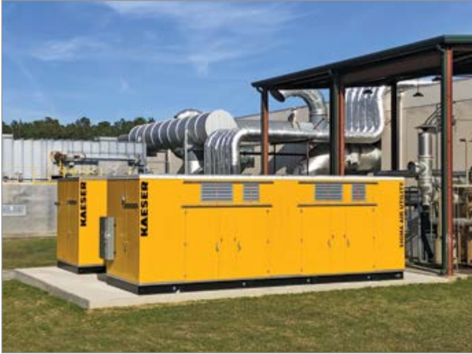
This 3,000 cfm compressed-air-as-a-service utility was delivered ready-to-run in two custom all-weather enclosures.
