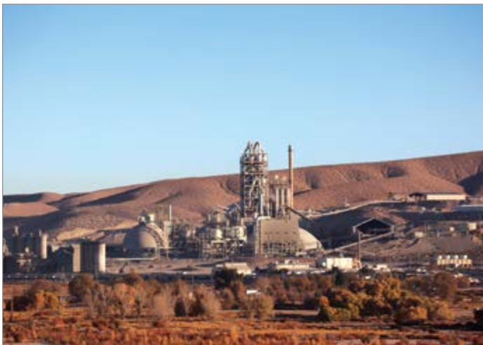
CalPortland operations, such as the company's cement plant in Oro Grande, CA, have long been recognized for success in sustainability.
