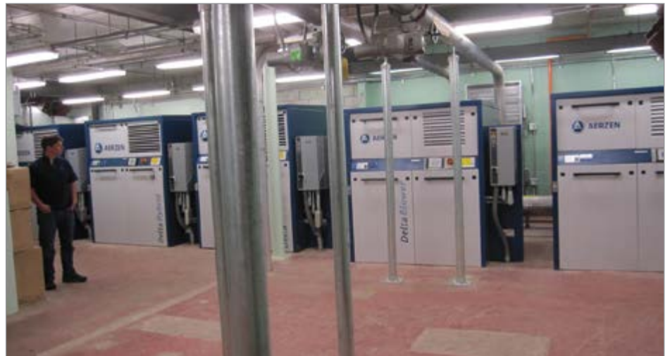
Hybrid and positive displacement blowers were housed together in a newly constructed blower room.
